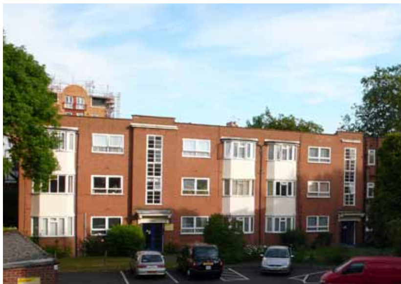
Above: evening light on back block – this is the only direct sunlight living rooms and some bedrooms receive. It will be considerably reduced by the proposed scheme (see page 3)
