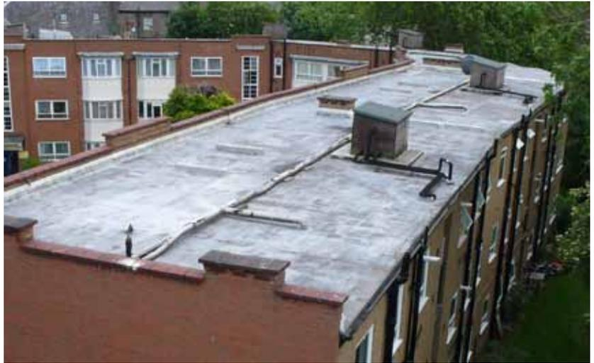
The tanks that feed all these flats are to be grouped at the north end of the back block (the nearest part of the roof here). They will have to be raised significantly to allow sufficient fall in the water; this will affect the roof line and the light received by the front block.
