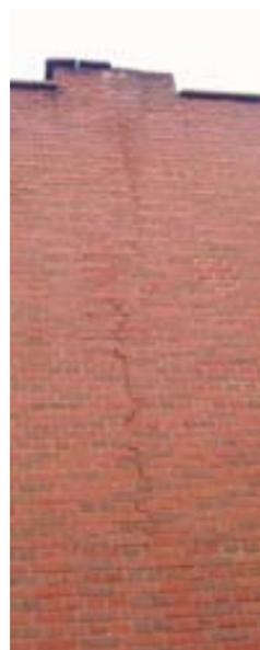
Crack in flank wall of back block
